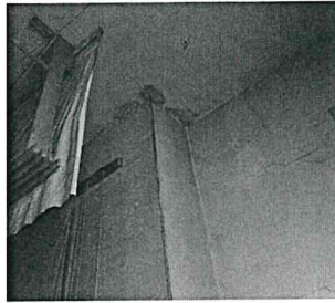
Chimney beside stage (Both sides)
