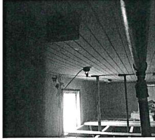
Under stage near back wall
