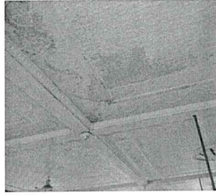
Ceiling above balcony
