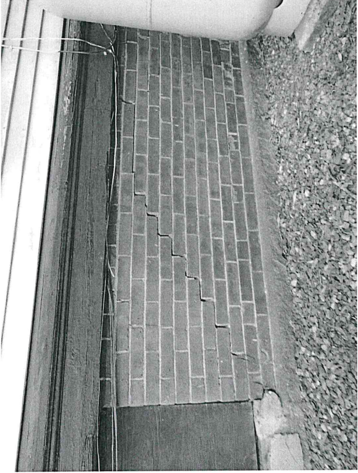
Foundation Crack
