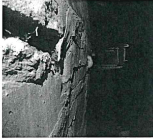
Basement wall on Parking lot side
