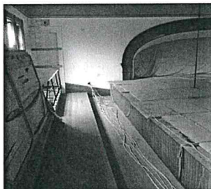
Electrical on Balcony floor
