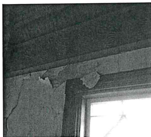
Balcony near windows
