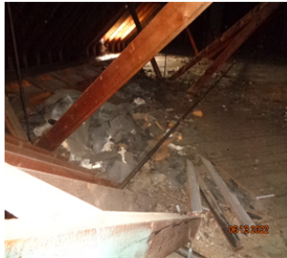
Attic pile of what appears to be slate shingles/ tiles for roof.
