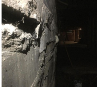
Basement wall on Parking lot side
