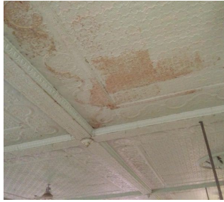
Ceiling above balcony
