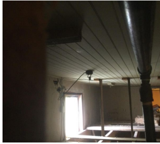
Under stage near back wall
