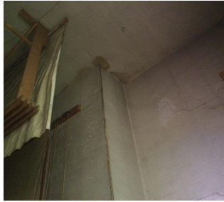
Chimney beside stage (Both sides)
