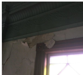
Balcony near windows
